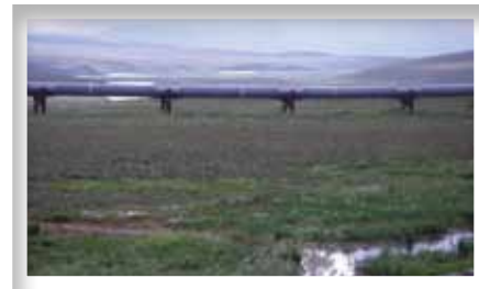
Trans-Alaska Pipeline between pump stations 2 and 3
