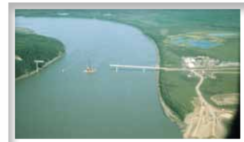
Yukon River Bridge construction. BLM Photo
