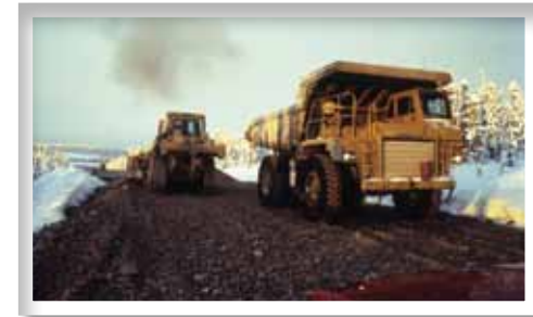
Building the TAPS Haul Road. BLM Photo
