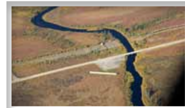
Dalton Highway crossing the Kanuti River— Trans-Alaska Pipeline dips underground Photo by Steve Hillebrand/USFWS
