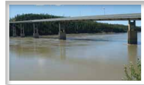
Yukon River Bridge, milepost 56
