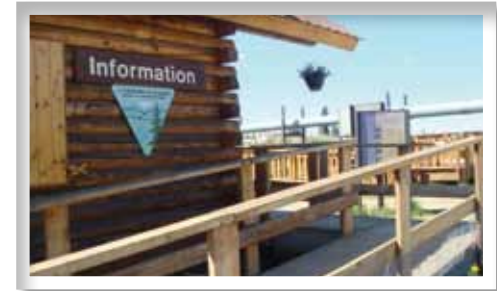
BLM Visitor Contact Station at the Yukon River Crossing, milepost 56—Trans-Alaska Pipeline and Yukon River Bridge in background
