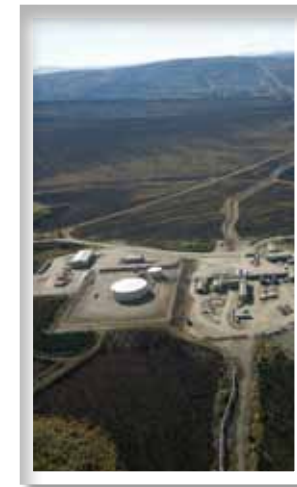
Pump Station 5 Photo by Steve Hillebrand/USFWS
