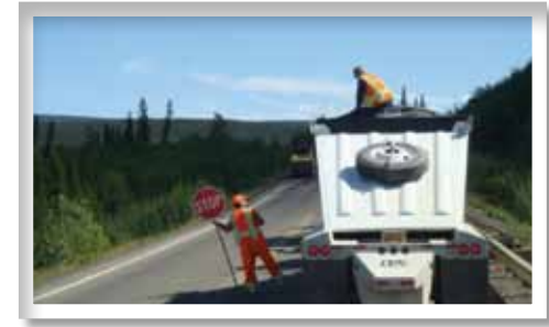
Road construction north of Livengood
