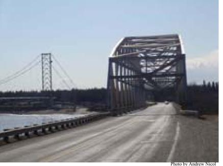
built to withstand an earthquake measuring up to a magnitude of 7.5 and temperatures as low as -60 degrees Fahrenheit.
