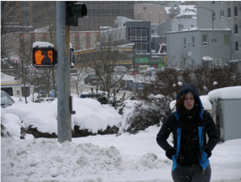
Pedestrian countdown timers were selected as a new standard safety feature in 2007. Many existing crosswalks will be equipped beginning in 2008. Photo Credit: Robert Laurie, Alaska DOT&PF
