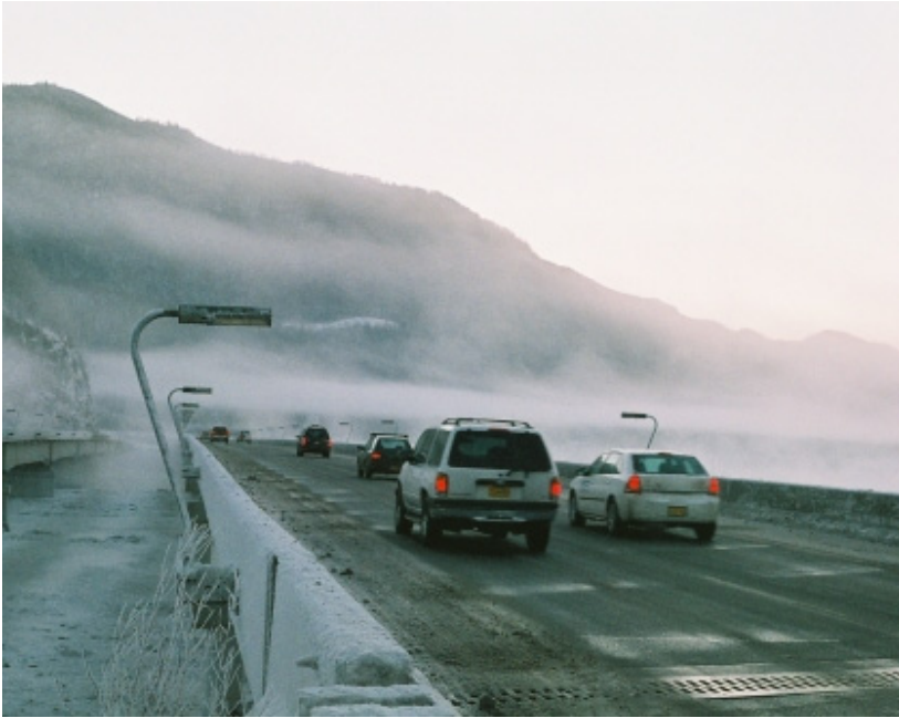
Glenn Highway bridge at Knik River, where an anti-ice system was recently installed.
