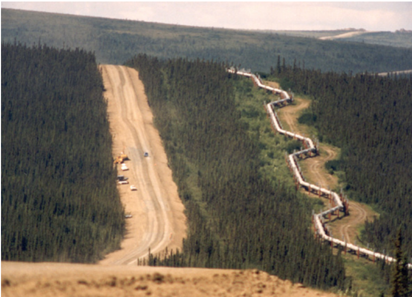
Dalton Highway alongside the pipeline (in 1994) Photo Credit: © Oscar Voss
