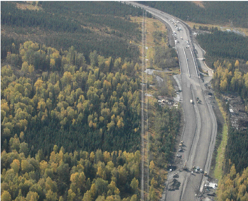
Elmore Road (Abbott Loop Extension) opened in 2007, several years sooner than a federally funded project would have been possible. Photo credit: Kurt Hutleen and Brian Hanson, DOWL Engineers.
