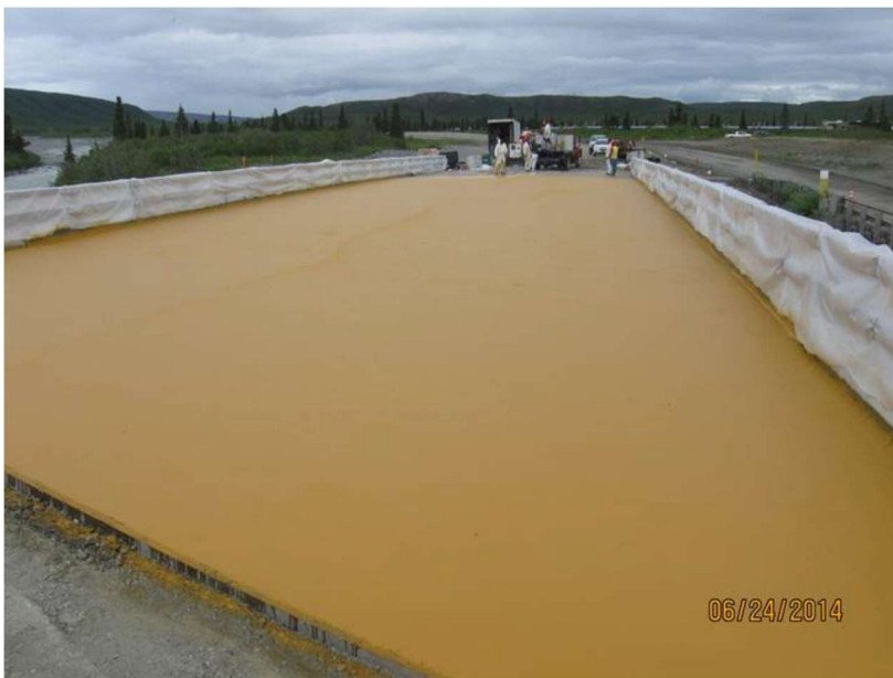
Figure 2: The first layer dries within 28 minutes but remains tacky for much longer. The second layer was started around 10 PM but was delayed due to rain. The first and second layers are identical in chemistry, only the color is different to ensure another complete 60 mil coat.
