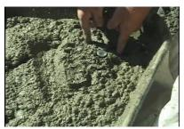
Pressing concrete around sensing device
