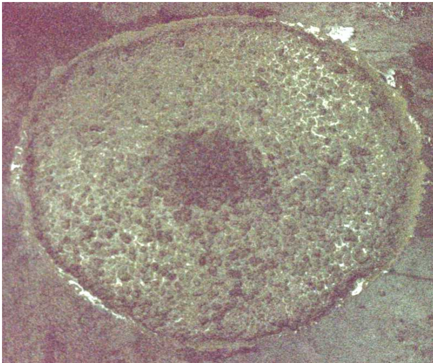
VSI 3: Unstable mix, visible halo around edges, segregation in middle, excessive bleeding.
