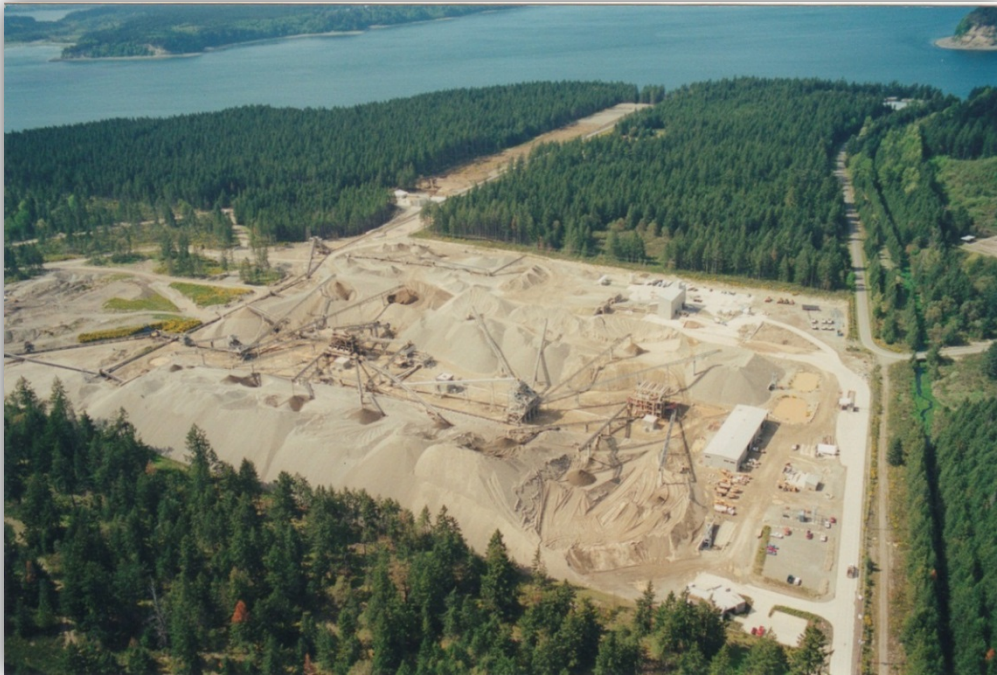
FIGURE 9 CALPORTLAND PIONEER AGGREGATE PLANT
