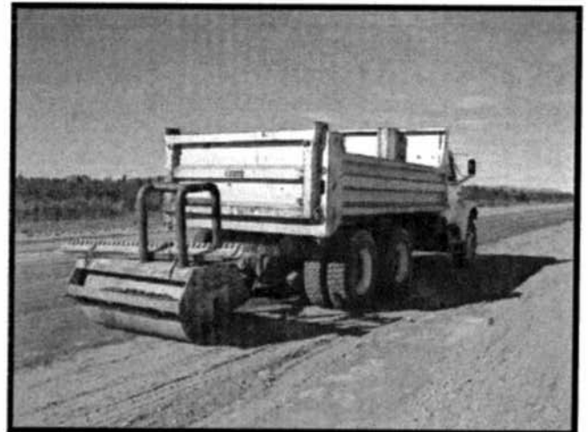
Photo 8: Compacting Runway
