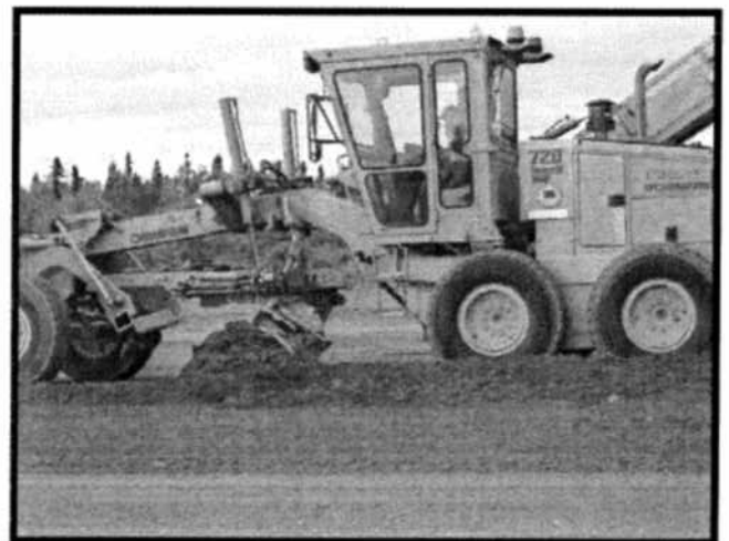
Photo 4: No Visible Dust Emissions During Grading
