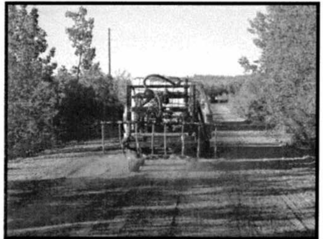
Photo 12: Applying Palliative on Airport Road
