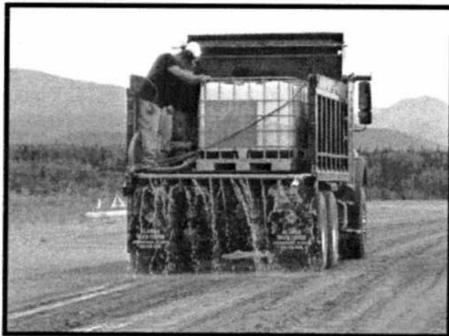
Photo 7: Applying Water to Runway
