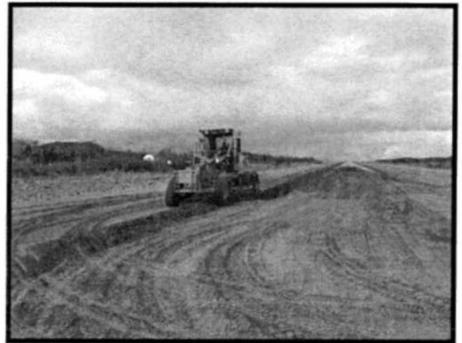
Photo 2: Grading Runway
