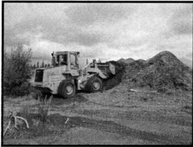
Photo 1: Loading Gravel at Quarry
