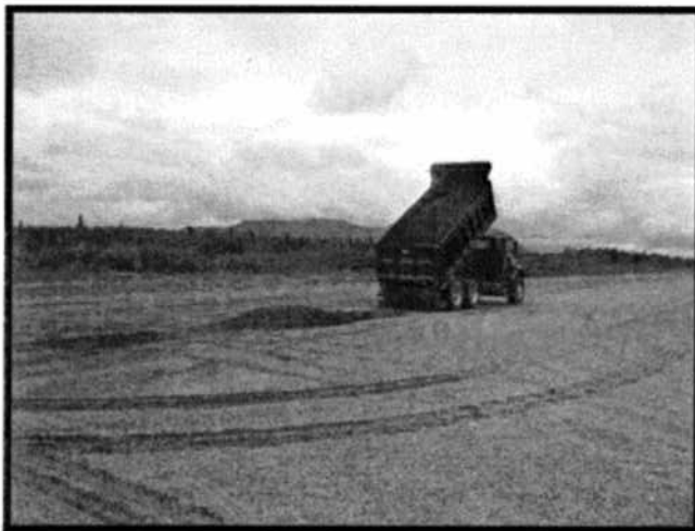
Photo 3: Spreading Gravel on Runway
