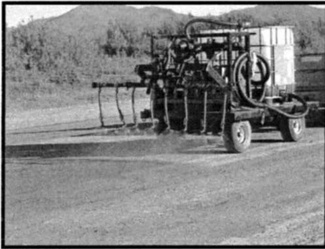
Photo 9: Applying Palliative on Runway
