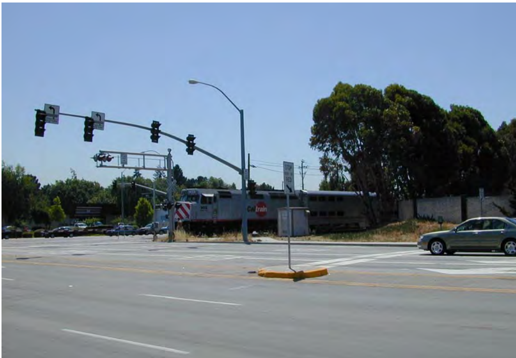
Figure 51. Pre-Signal Located Ahead of Grade Crossing with Displaced Stop Bar, S. Mary and W. Evelyn at Caltrain Commuter Line, Sunnyvale, California
