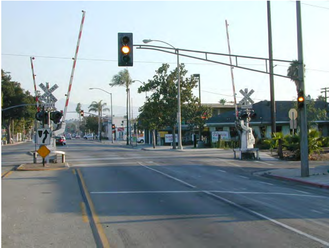
Figure 53. Queue Cutter, Magnolia Street at Union Pacific Railroad, Riverside, California
