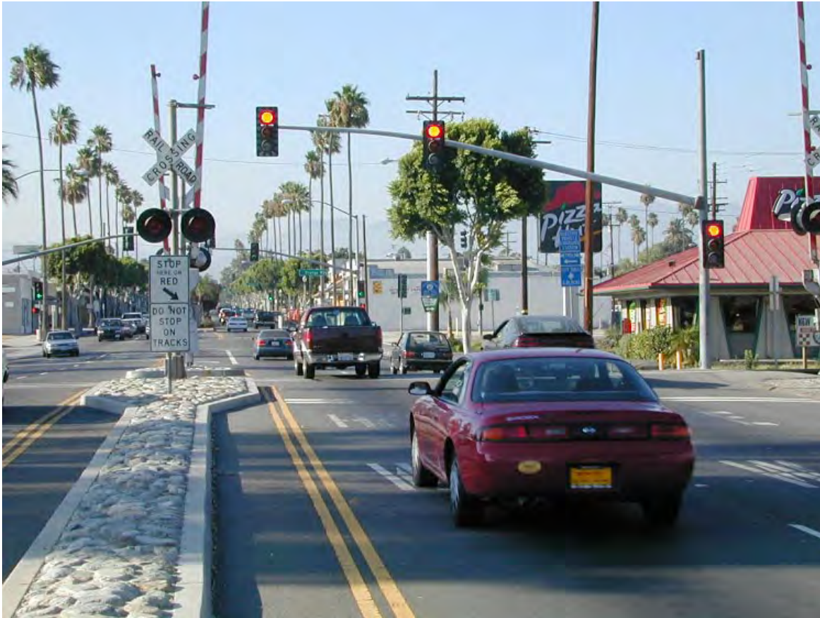
Figure 52. Pre-Signal with Louvered Downstream Intersection Signal, Sierra and Orange at Metrolink Commuter Line, Fontana, California
