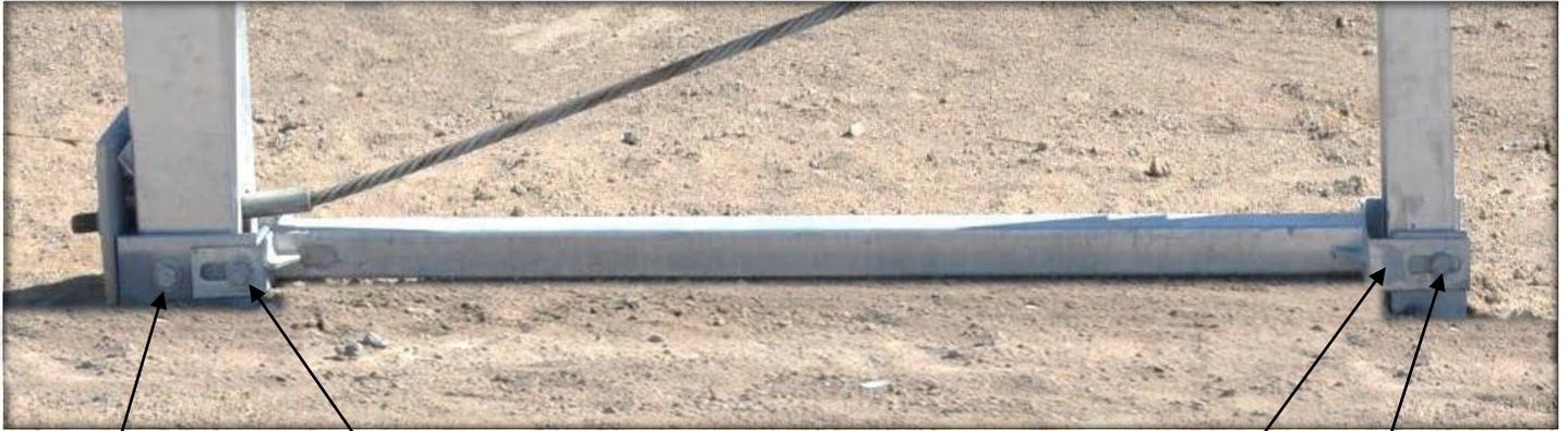
5/8" x 9" hex bolt, nut, & washer at post #1 on upstream side of the post
