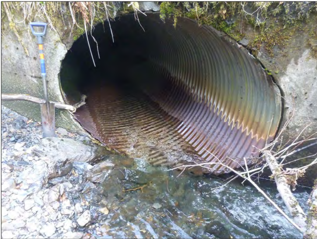
Site 594: Downstream view of stream to culvert inlet. Photo taken May 7, 2018.
