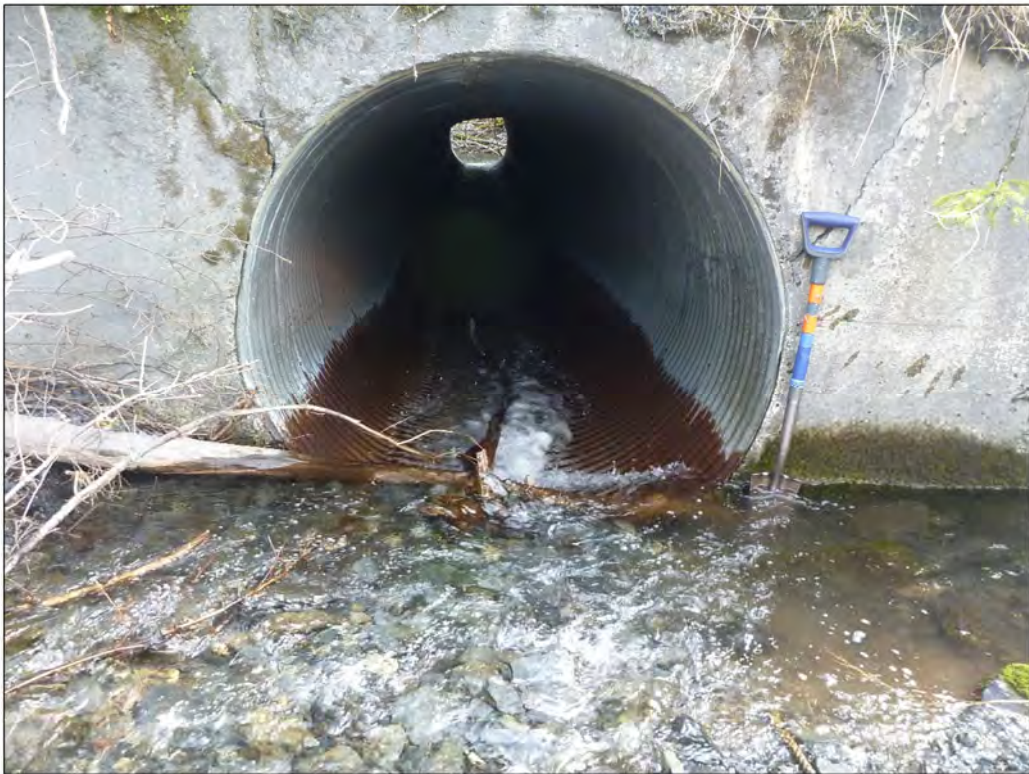
Site 593: Downstream view of stream to culvert inlet. Photo taken May 7, 2018.
