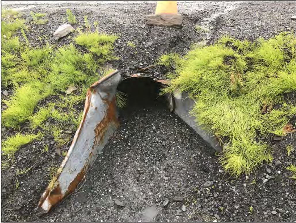
Site 041: Culvert outlet. Photo taken July 24, 2018.
