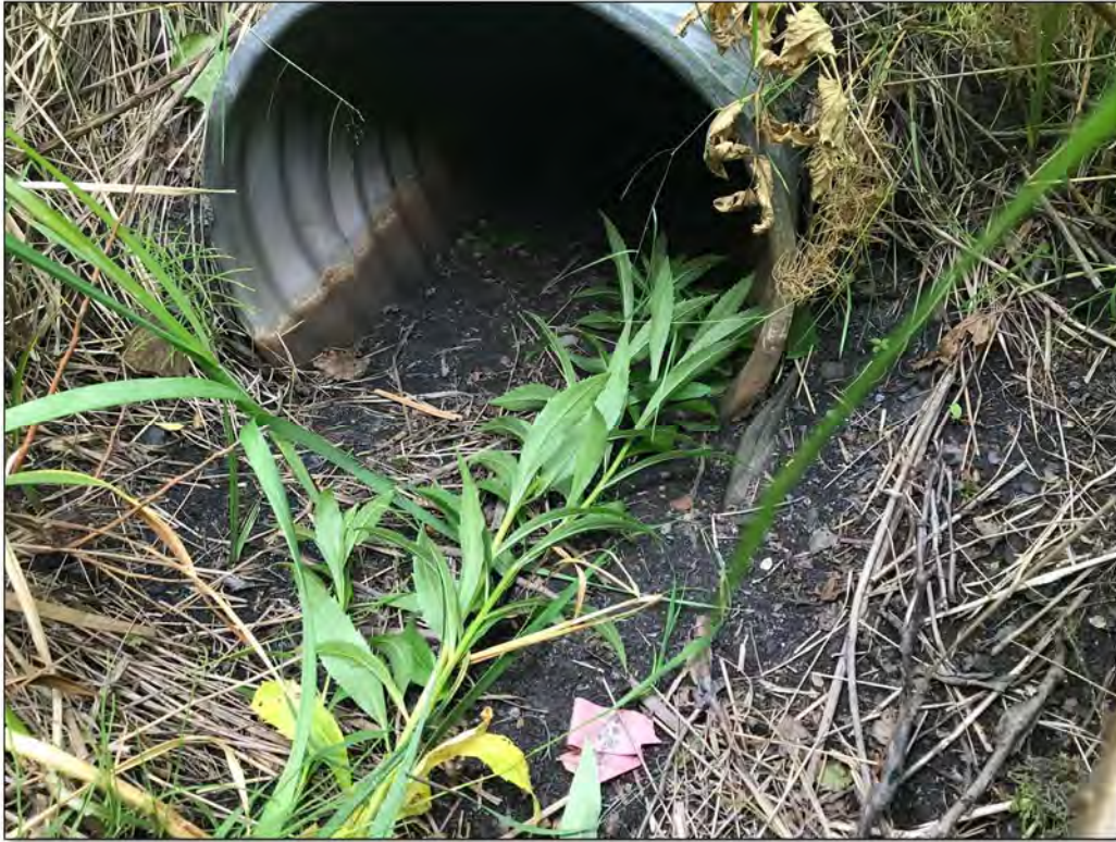
Site 008: Culvert outlet. Photo taken July 19, 2018.
