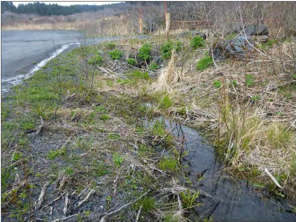
Site 574: Downstream view of stream to culvert inlet. Photo taken May 7, 2018.
