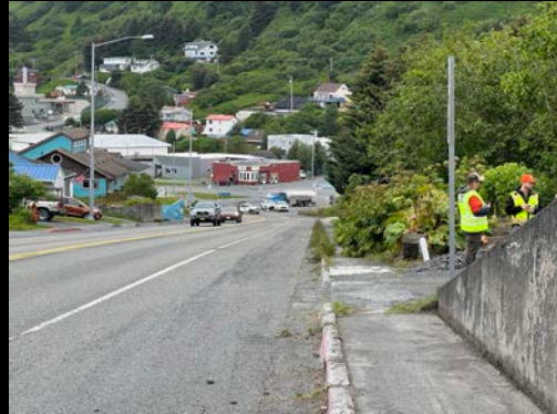
Steep Sidewalks at Driveways
