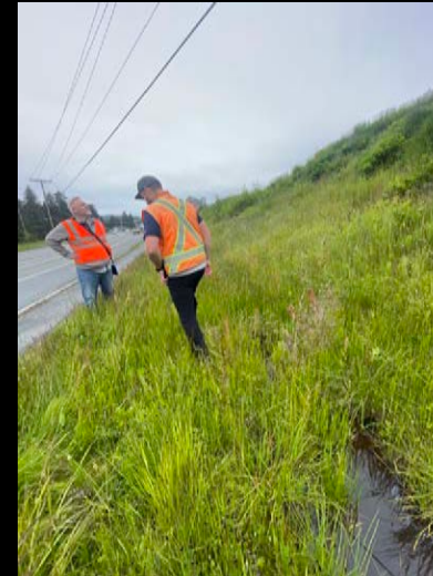
Ditches Draining onto Sidewalks
