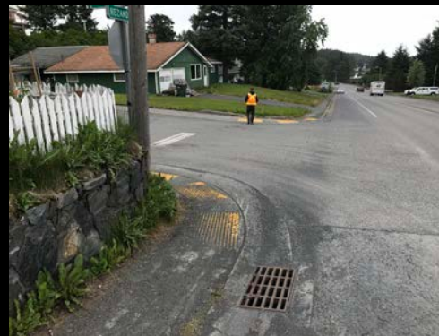
Light Poles Restricting Sidewalk Space
