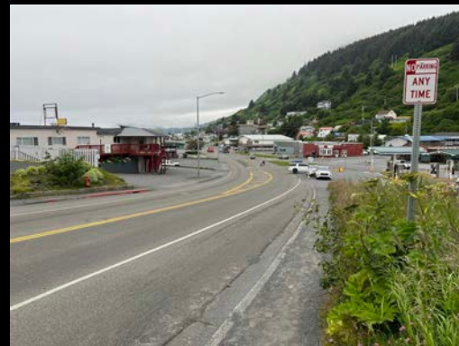
Overgrown Vegetation Limiting Sidewalk Width
