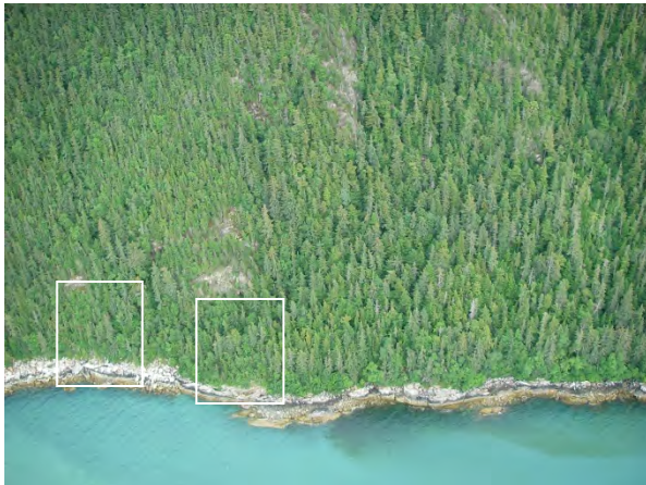
RF43 & RF44. View east/upslope at rockfall areas RF43 (right) and RF44 (left).
