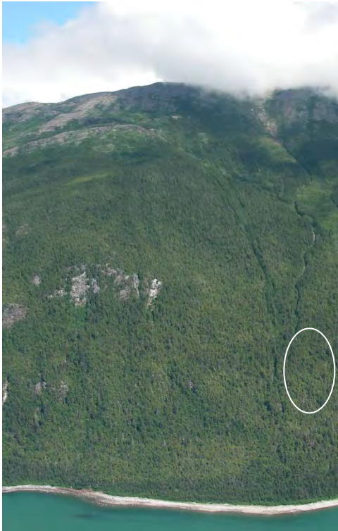
RF12. View east/upslope at rockfall area.
