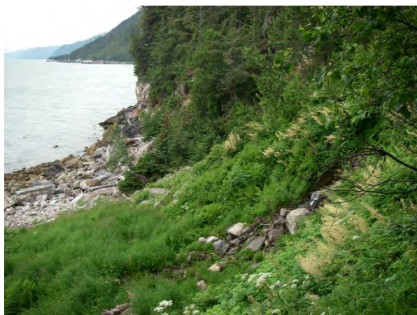
DF28. View northwest (up alignment and downslope) at deposition fan of debris flow.
