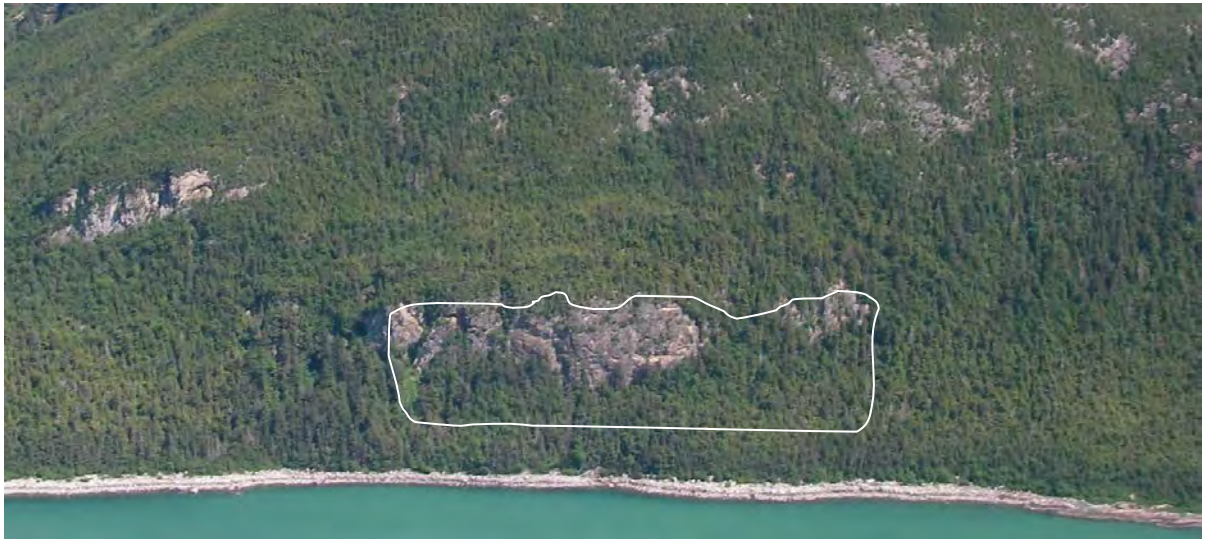
RF14. View east/upslope at moderate rockfall hazard below massive gneiss cliffs.
