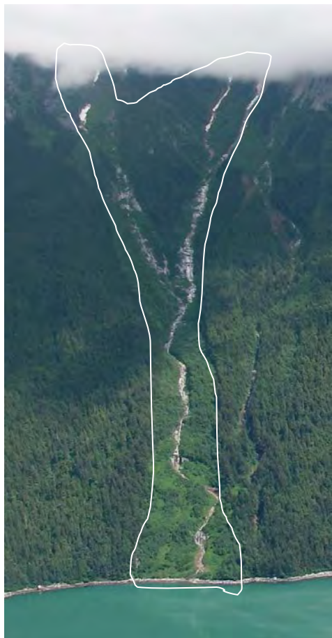
DF26. View east/upslope at debris flow channel and avalanche path.
