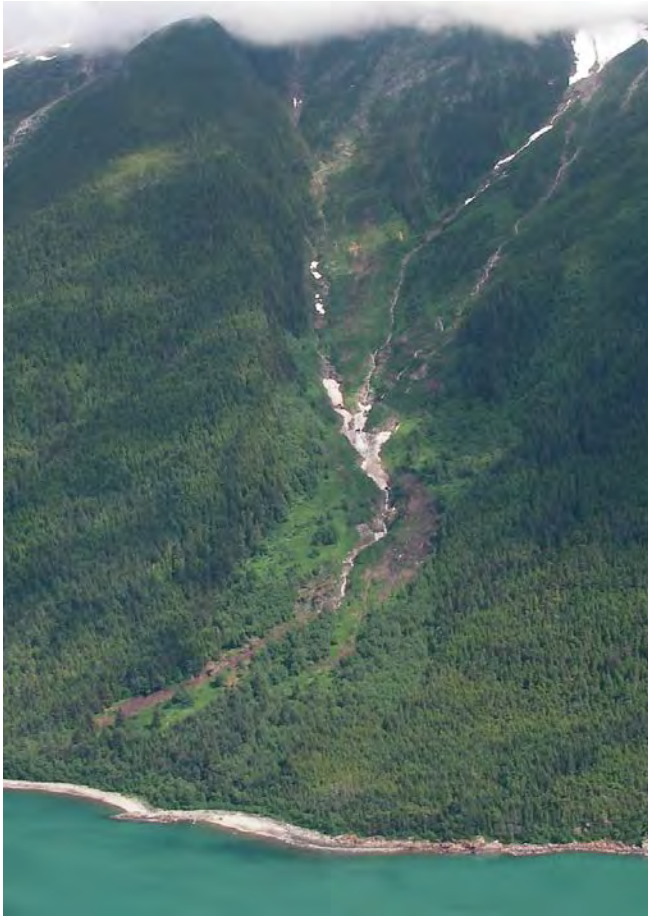
DF18. Debris flow and avalanche path.
