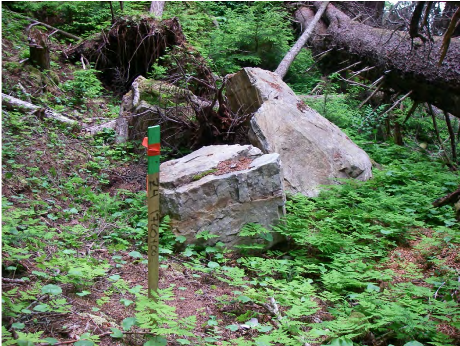
RF08. View southwest (downslope and down alignment) at rockfall debris. Survey lath represent previous IRP 2006 alignment.
