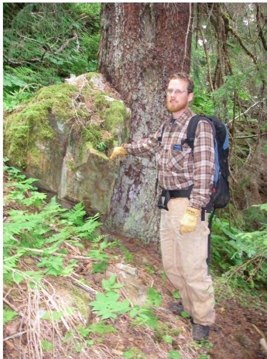
RF41. View south/down alignment at rockfall stopped by a spruce tree.
