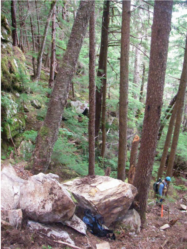
RF45. View west/downslope at rockfall with fresh rockfall stopped by spruce trees.
