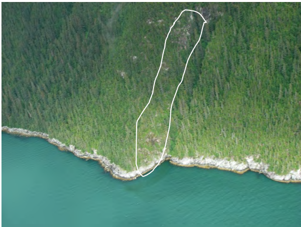
RF28. View east/downslope at rockfall hazard area.
