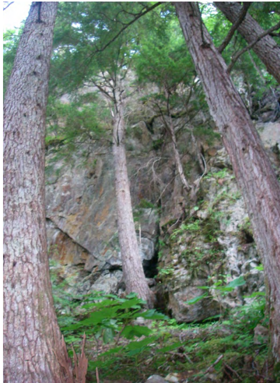
RF47. View east/upslope at rockfall.
