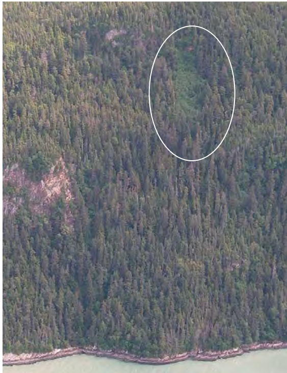
LS06. View east/upslope at landslide area (green patch of disturbed vegetation in upper right photo).
