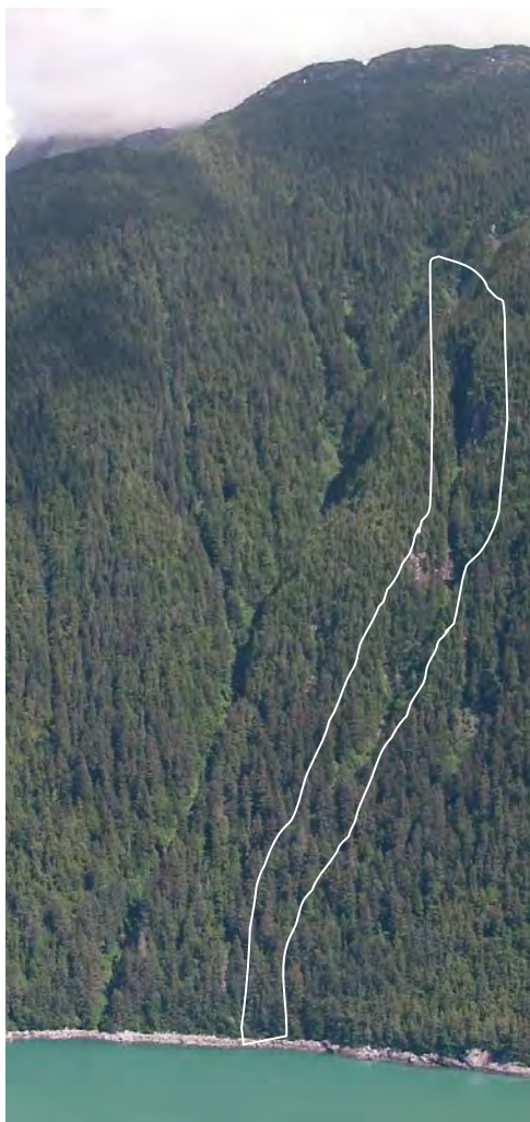
RF31. View east/upslope at rockfall hazard and avalanche path.
