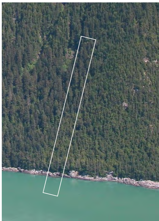
RF30. View east/upslope at rockfall hazard.
