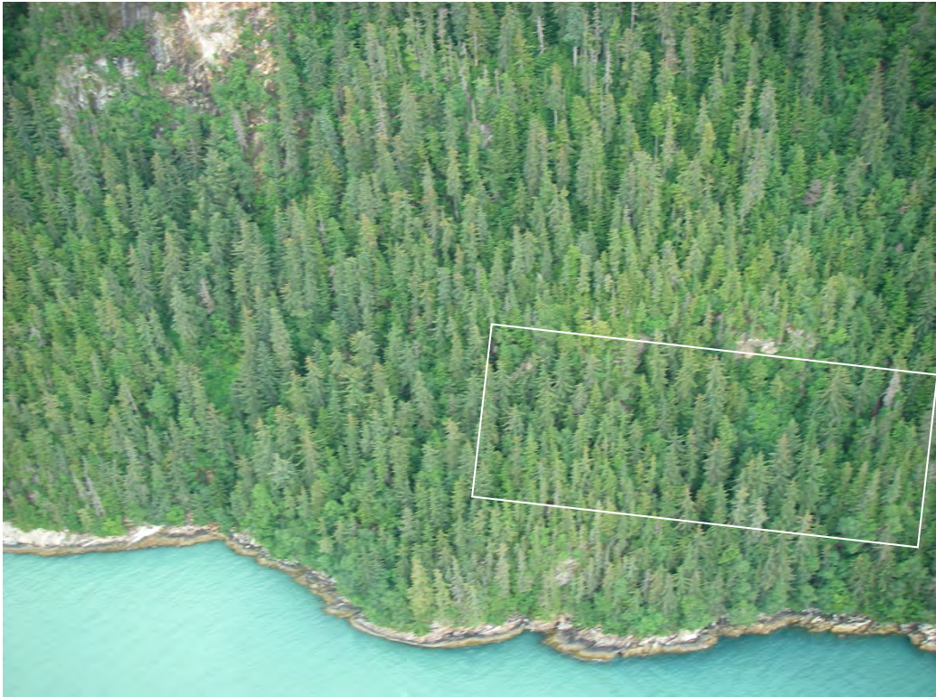
RF47. View east/upslope at rockfall hazard area.
