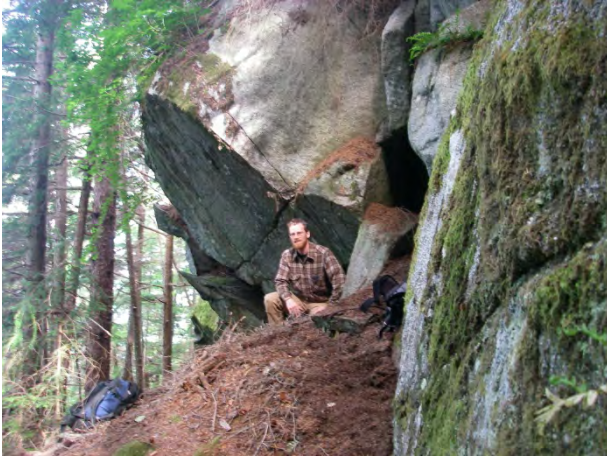
RF26. View north/up alignment at rockfall hazard.
