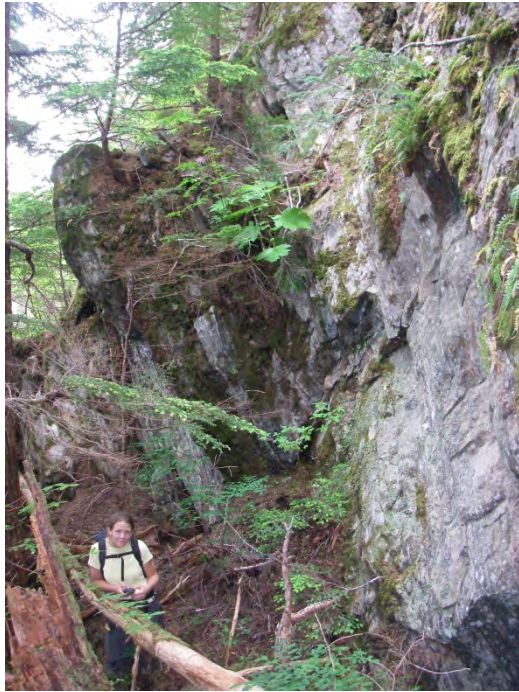
RF21. View north/up alignment at rockfall hazard.
