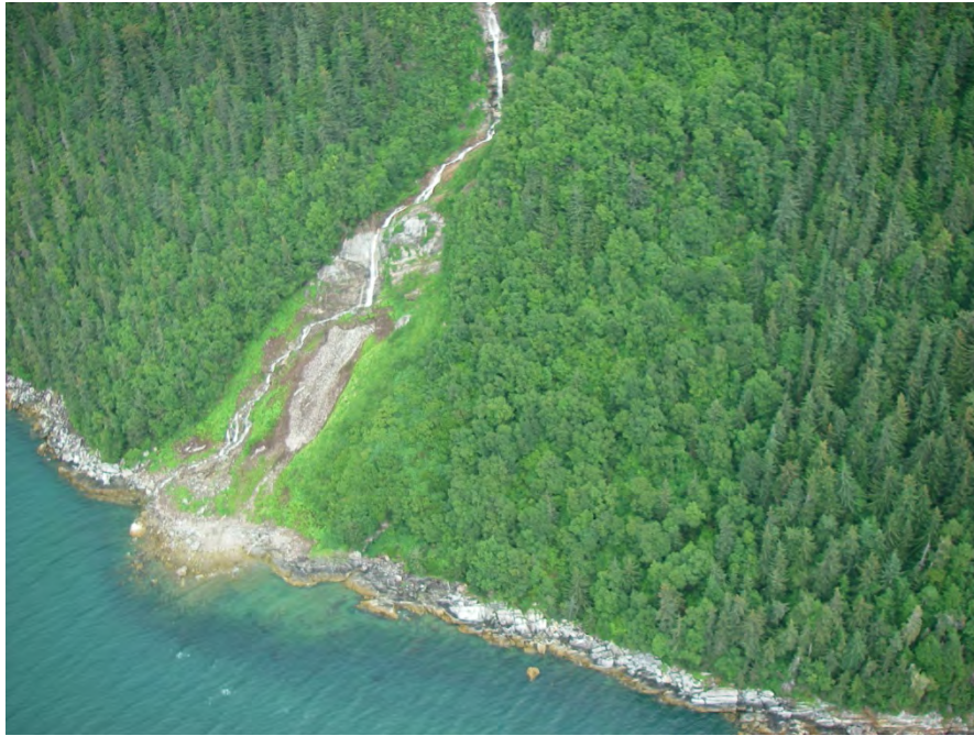
DF29. View northeast (up alignment and upslope) at debris flow deposition zone and avalanche path.
