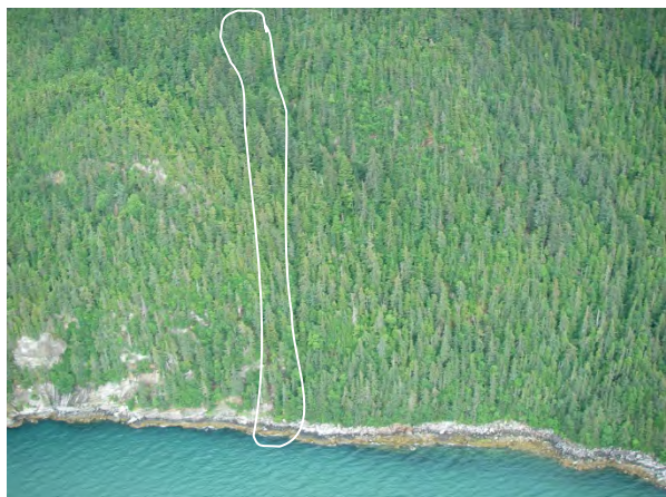
RS02. View east/upslope at rockfall hazard and rockslide.
