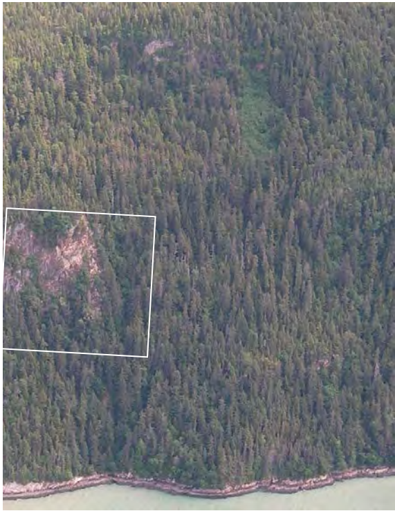
RF49. View east/upslope at rockfall hazard below cliffs.
