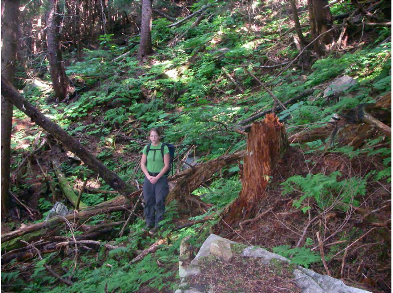
RF16. View north/up alignment across low frequency rockfall area.
