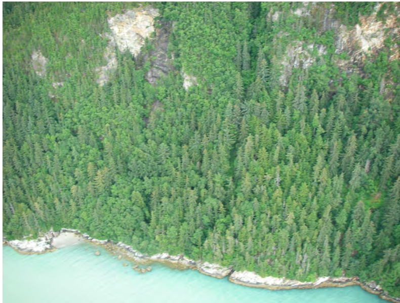
RF49. View east/upslope at the north half of rockfall area.
