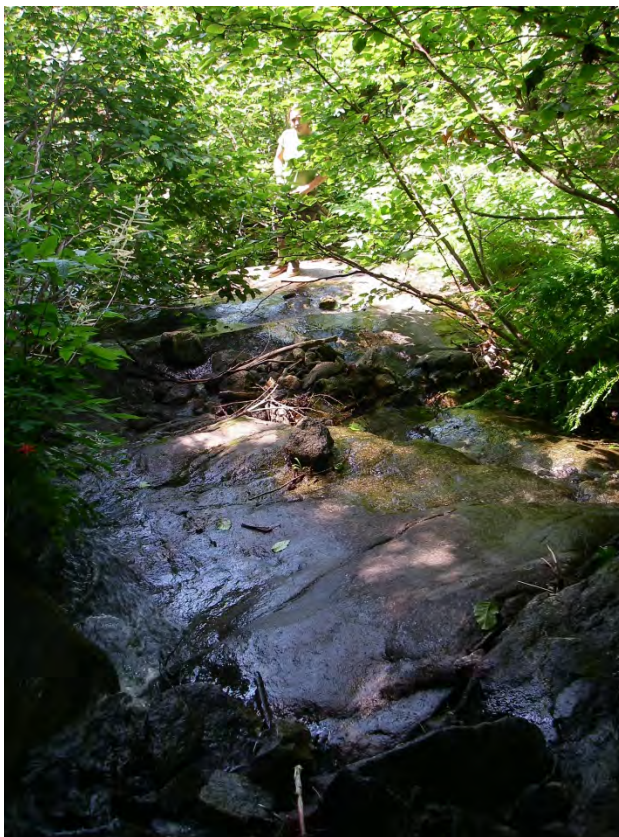
DF36. View west/downslope at debris flow channel scoured to gneiss bedrock.
