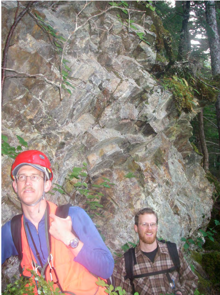
RF24. View east of rockfall hazard with fresh scarring.
