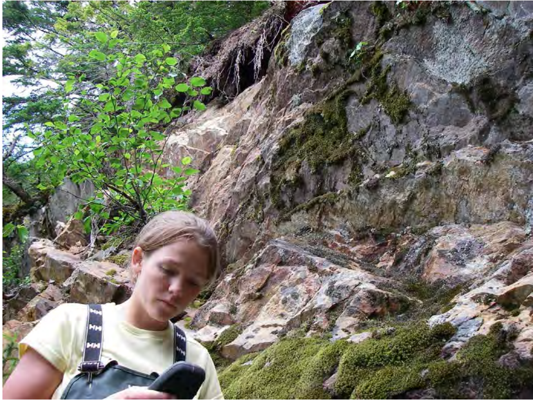
RF10. View at basalt cliffs that create the rockfall zone.
