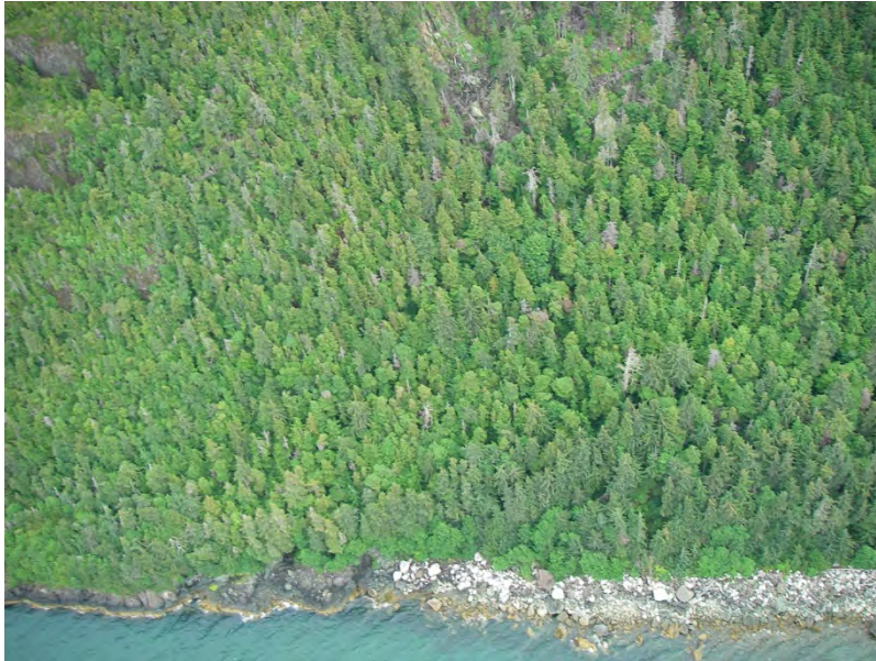
RS01. View east/upslope of area directly under rockslide. Some debris approaches the 2012 SEIS alignment which is located just east/upslope of the beach.
