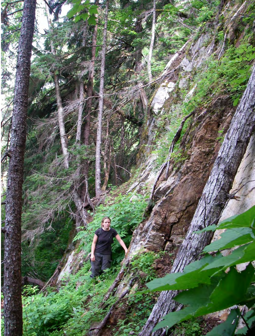
RF51. View north/up alignment across steep face of rockfall hazard.
