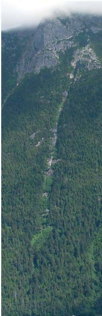
RF17. View east/upslope at rockfall hazard area.
