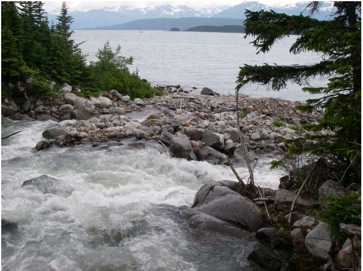
DF22. View southwest (downslope and down alignment) at debris flow fan and avalanche path.
