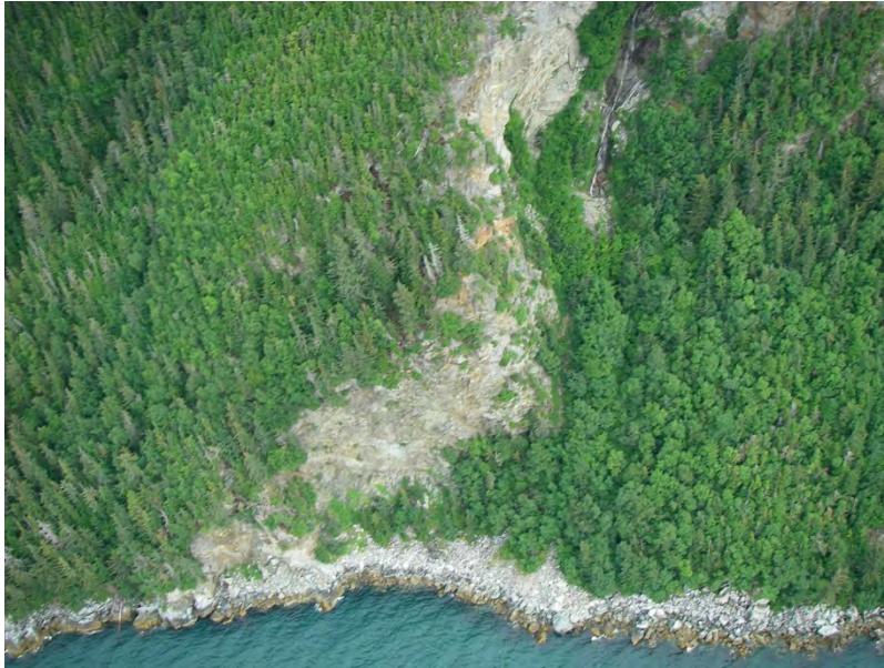
RF07. View east/upslope at 500 ft high gneiss cliffs with strong jointing and rockfall.
