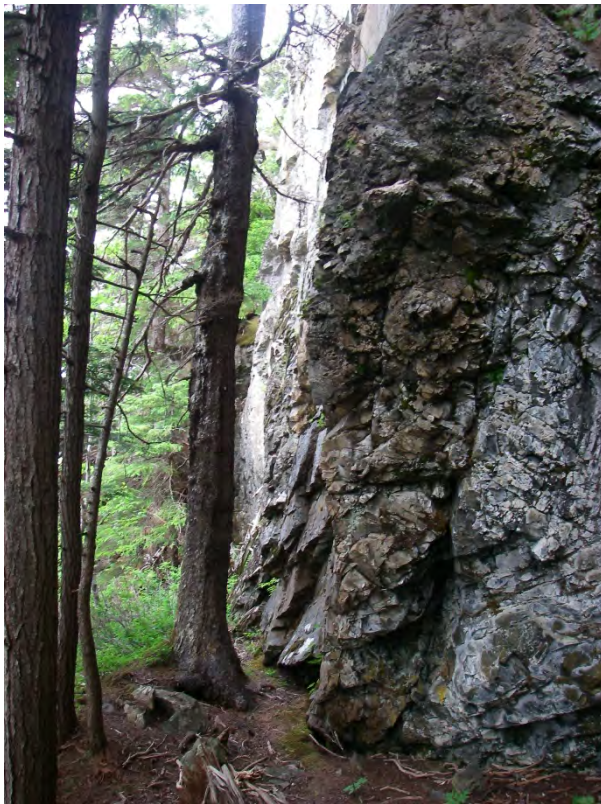
RF04. Base of vertical basalt cliff creating rockfall hazard.
