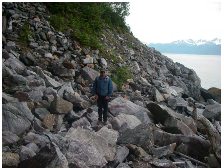
DF09. Debris flow and talus cone at base of debris flow and avalanche path.
