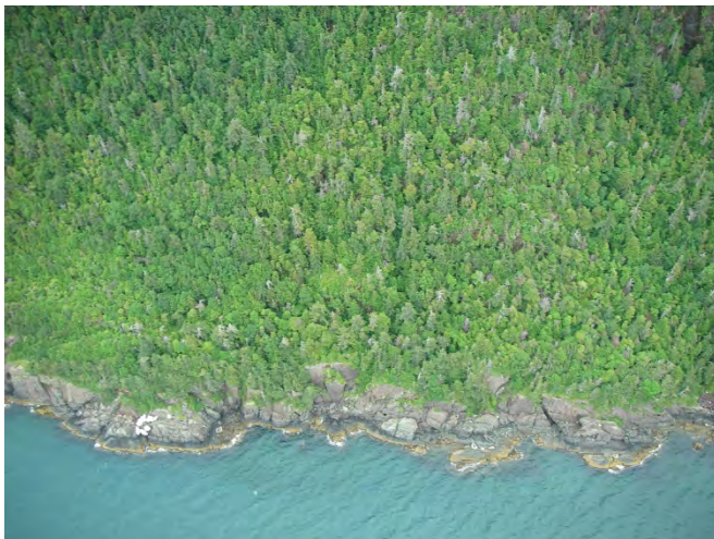
RF03. View east/upslope at rockfall area.
