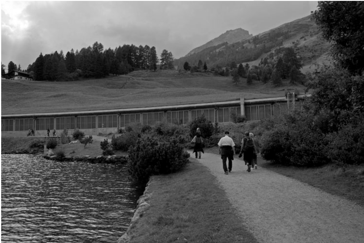
Figure 15: Shed-roof Gallery Snowshed, Davos, Switzerland
