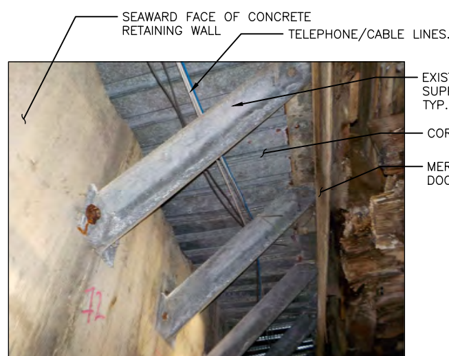
1 PHOTO: EXISTING BRACKET-SUPPORTED SIDEWALK SCALE: NOT TO SCALE
