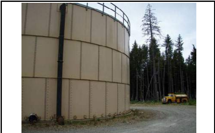
Community Water Tower
