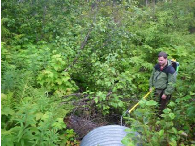
Figure 2.—Mr. Rick Hoffman downstream of stream 10A culvert.
