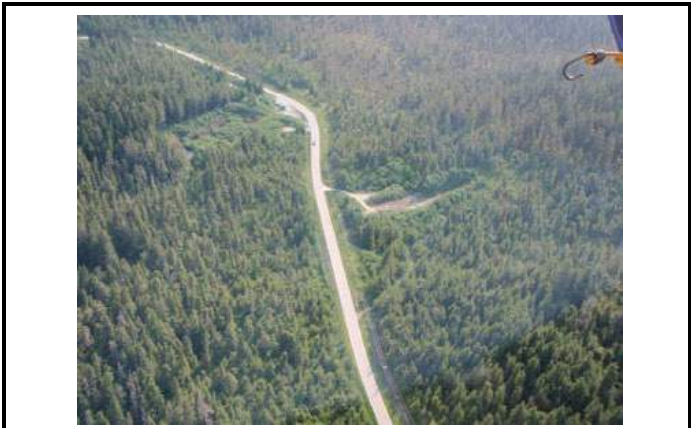
Road to Ferry Terminal and Landfill
