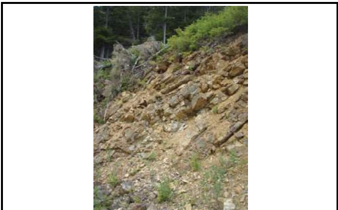
Cut on near Water Tower
