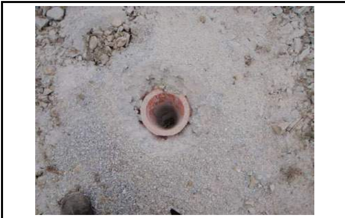
Drilled Holes Covered with a Cone at the Existing Gravel Pit
