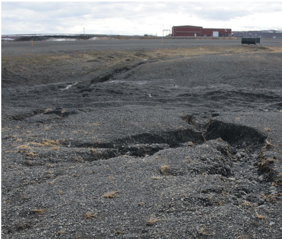
Graphic 4: Current Drainage Deficiencies on Runway 17/35
