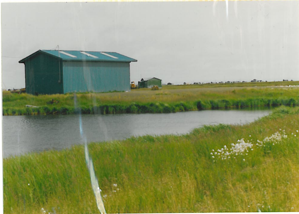
Looking southeast at old borrow cell and Maintenance & Operations building on the existing apron from Sta. 15+00.
