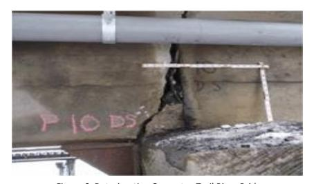
Figure 6. Deteriorating Concrete Trail River Bridge
