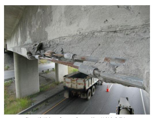
Figure 13. Highway Overpass Damaged by a Vehicle Collision
