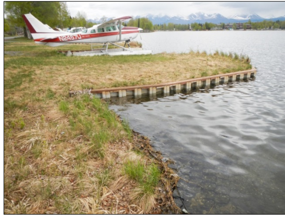
Floatplane Slip With Erosion Control in North Lake Spenard
